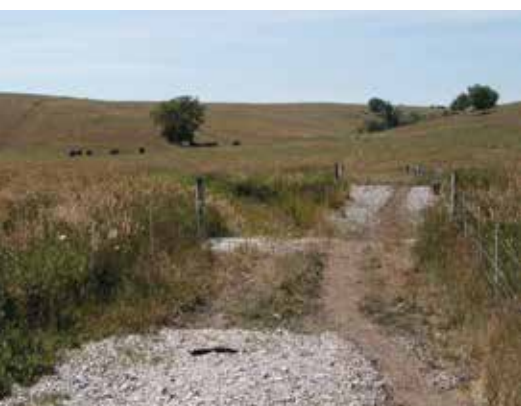
To minimize down-slope erosion, small diagonal berms can be formed in lanes to divert surface flow into adjacent pastures or buffers. Photo by James Russell.
