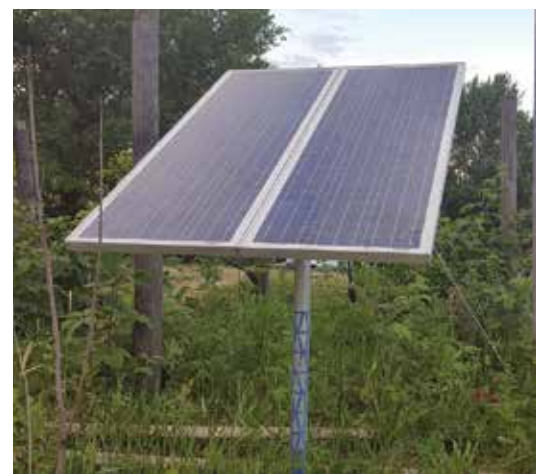
Solar pumps are effective at providing water to grazing cattle in remote locations. Photo by Denise Schwab.
