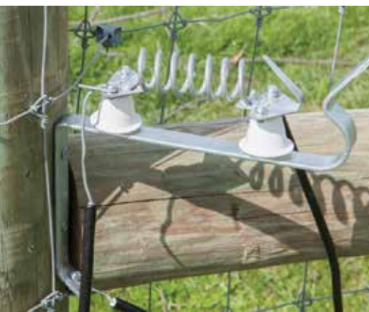
Lightning strikes along the electric fence line can damage the fence energizer. Use a lightning choke, as shown here, or another form of lightning protection. Photos by Samantha Jamison.
