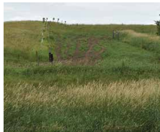
Frequent lane use and poor layout design lead to excessive erosion problems. Photo by Samantha Jamison.
